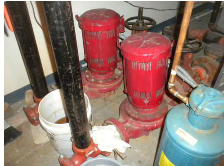
Two 7.5 horsepower pumps
