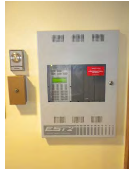
The central fire alarm control panel
