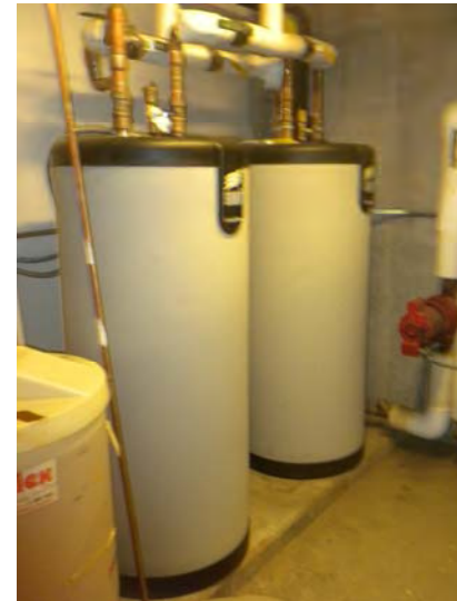
Triangle tube storage tanks
