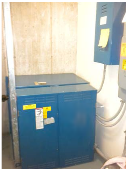
Hydraulic elevator equipment
